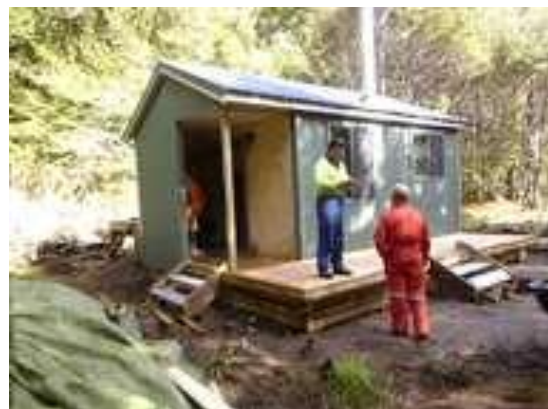
All finished - the new Maropea Forks Hut
