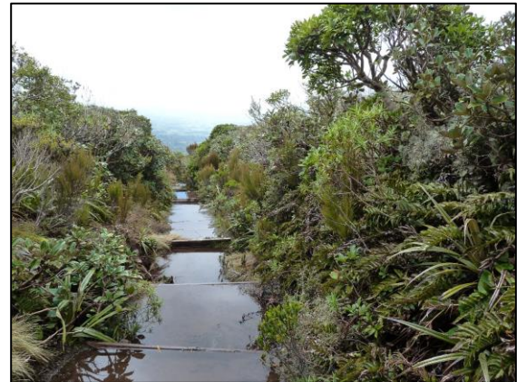
Waterlogged steps on Fanthams Peak track [Esther Pothuis]
