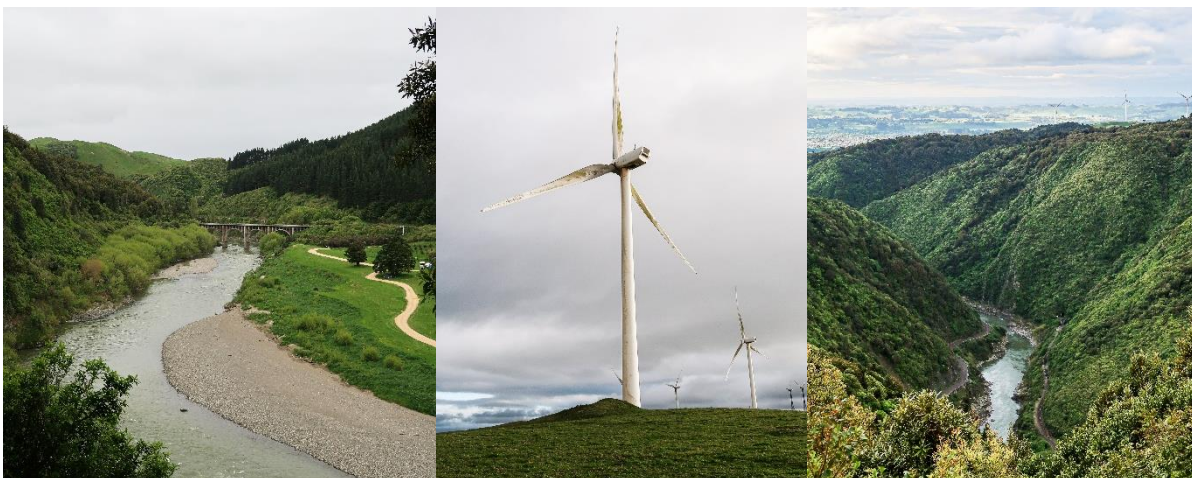
Views from Manawatu Gorge Walk route from Ballance end to Sentinel Lookout
