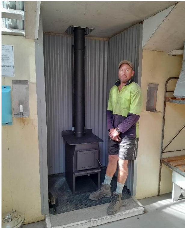
Chris Rayner with new woodburner installed.
